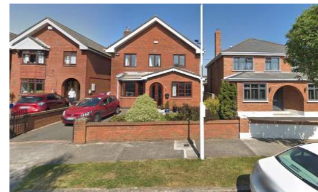
2 Storey houses on Willow Grove - Eastern Boundary
