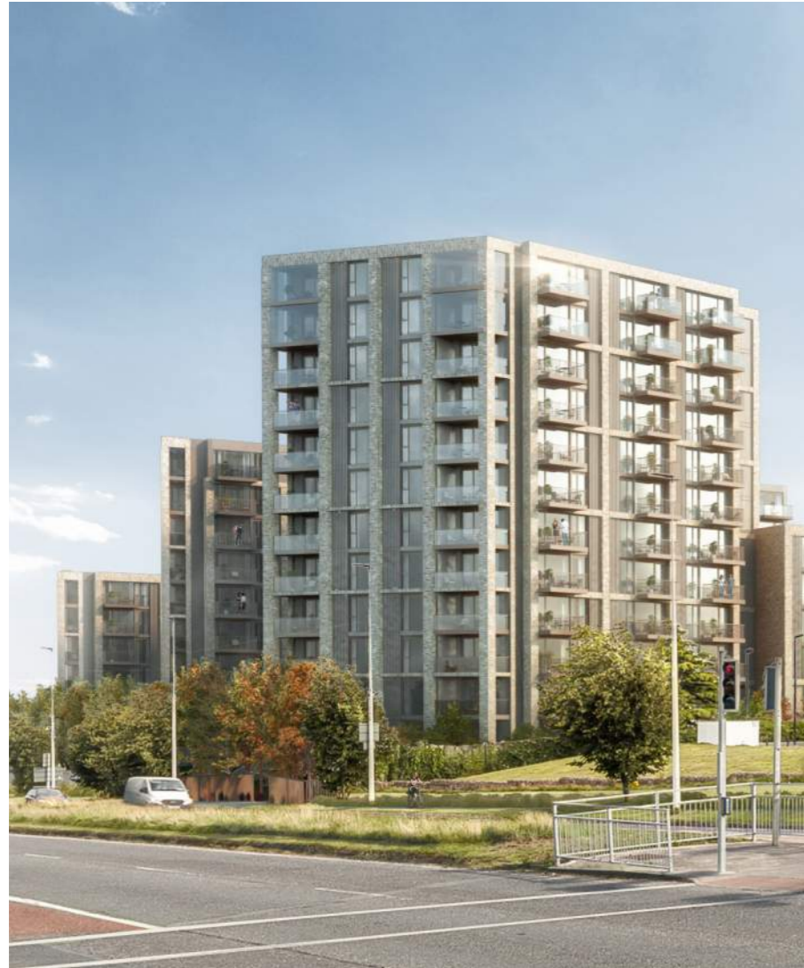
Buildings A,B & C - North Facing Facades
